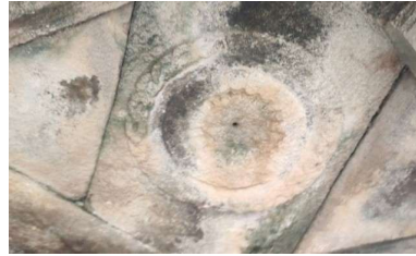
Figure 4: Chakra or round-shaped roof design with the serpents in a circular braid form, named K8 (Source: Author)
